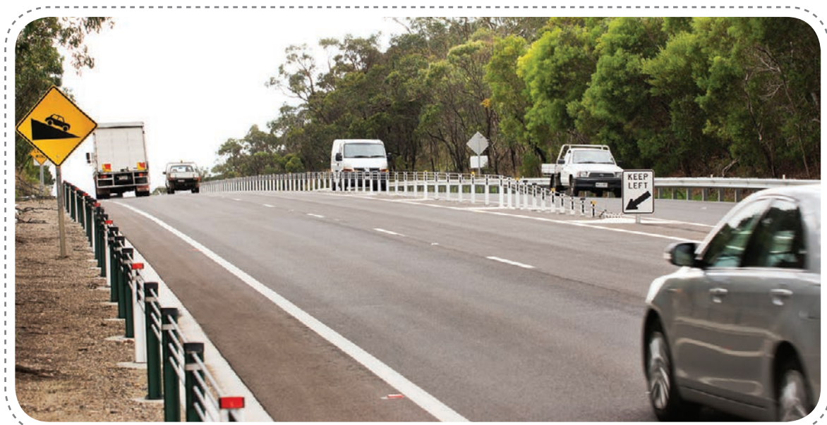
Wire rope barrier, Victor Harbor Road. Installed December 2012.
